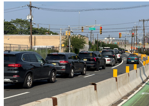
Jersey Avenue detour traffic
